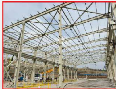
RÖNESANS Steel fabrication and installation works."
