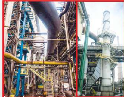
İSDEMİR VAGG – Manufacturing and installation of the dust collection system.
