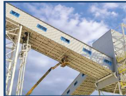
ŞİŞECAM – ANT YAPI Mechanical and steel fabrication and installation works.
