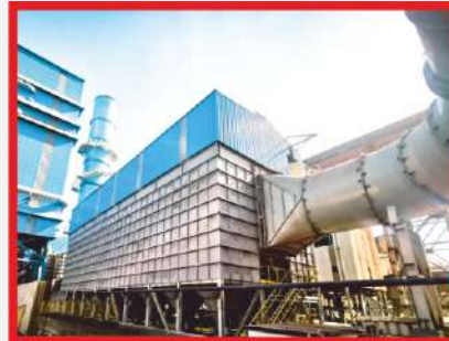
İSDEMİR 1. YF – Construction of dust collection systems.
