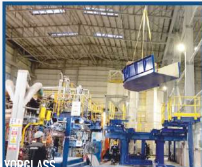
YORGLASS Glass plant construction and installation works.
