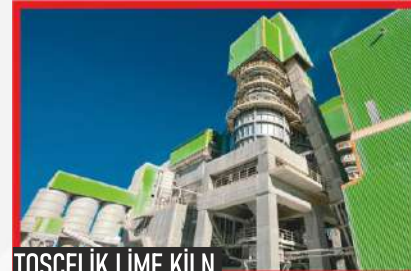
TOSÇELİK LİME KİLİN For the Tosyalı Plant, two lime plants with a capacity of 650 tons/day each and one dolomite plant with a capacity of 650 tons/day were manufactured and installed.
