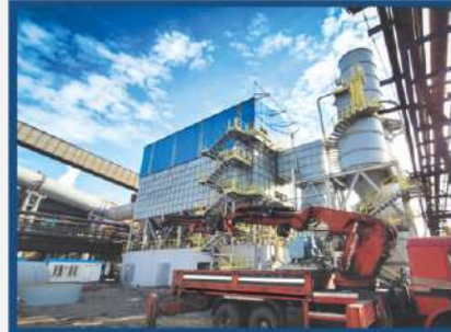
ERDEMİR Manufacturing and installation of the dust collection system were carried out.
